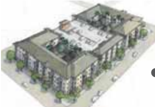
Example of multi-storey 'wrapped' car parking
